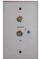
Antenna Power Supply
