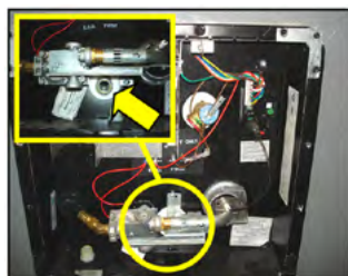
Water heater drain plug location
