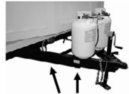
Electrical wiring & safety break-a-way switch
